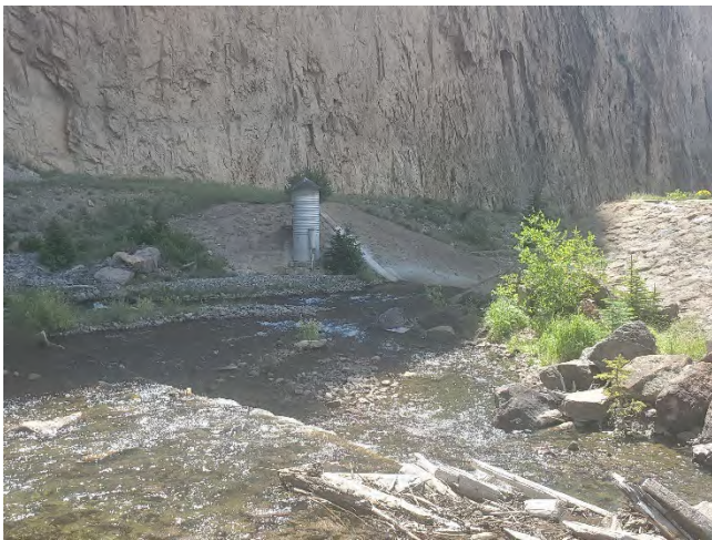
Photo 6. Willow Creek proposed location for Hydro Power Plant
